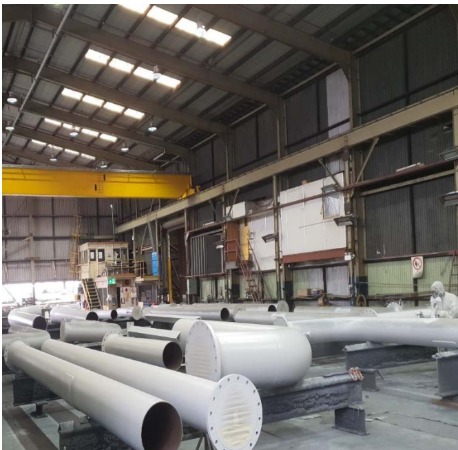
Prime Coating of Pipe Spools
