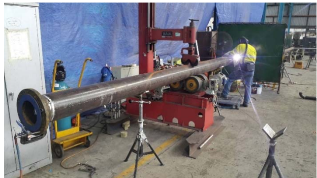
Cement Lined Piping for Gasoline Tank Proj
